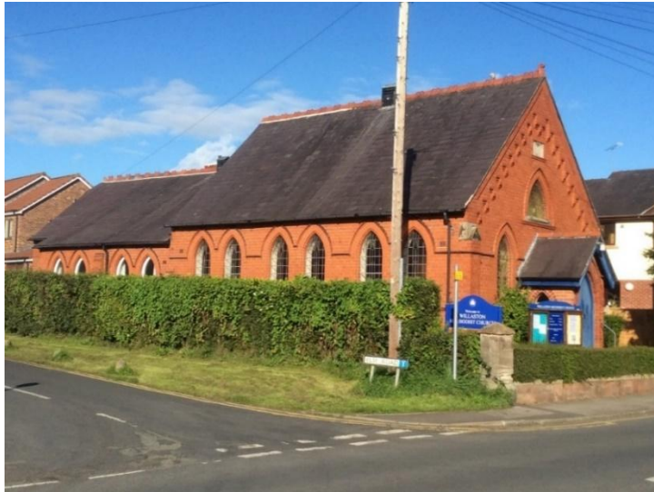
Willaston Primitive Methodist Chapel, built 1889
